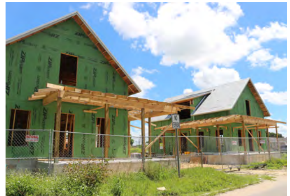
'Habitat for Humanity' Affordable housing construction on Center Street
