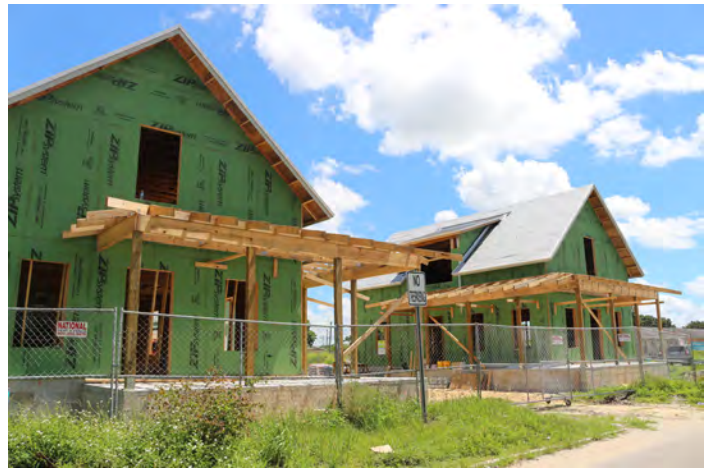
In-progress construction of Habitat Homes on Center Street
